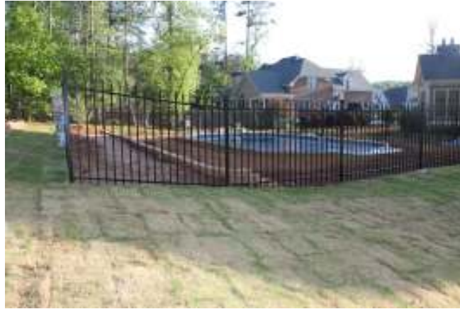
Pool barriers in unstable foundations!
