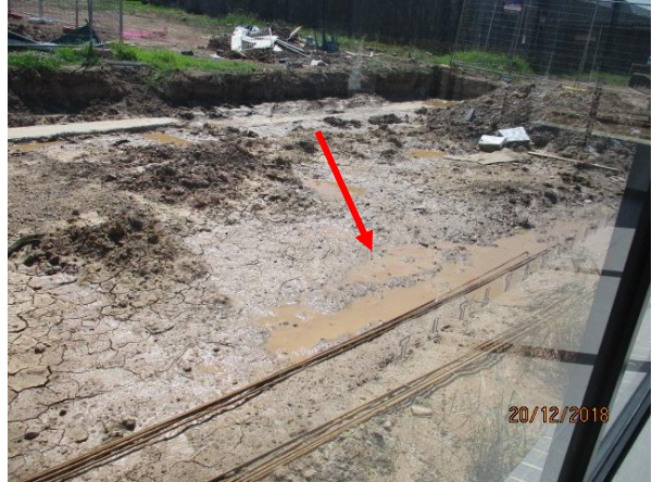
Cracking and crumbling due to inadequate site surface overland flow drainage
