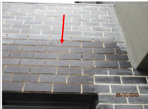
Blown out brickwork mortar joints
