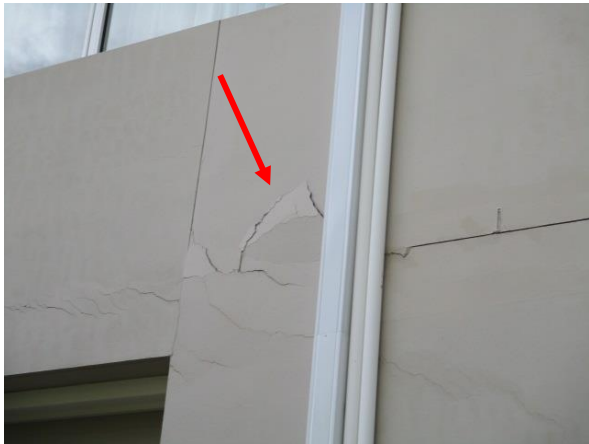
Cracking and crumbling due to inadequate site surface overland flow drainage
