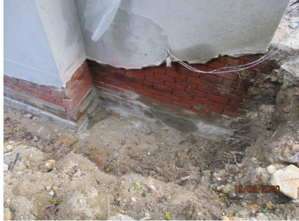
Moisture ingress due to inadequate waterproofing methods
