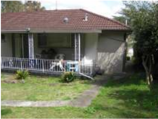
Granny Flat unit/As Inspected.
