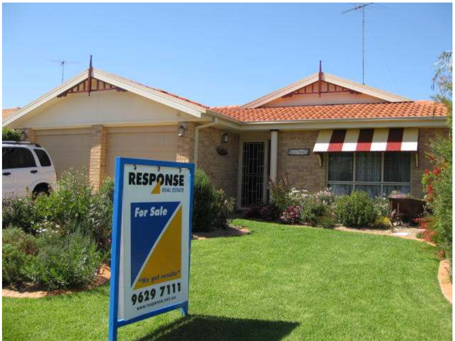
Front Elevation of the Inspected Property
